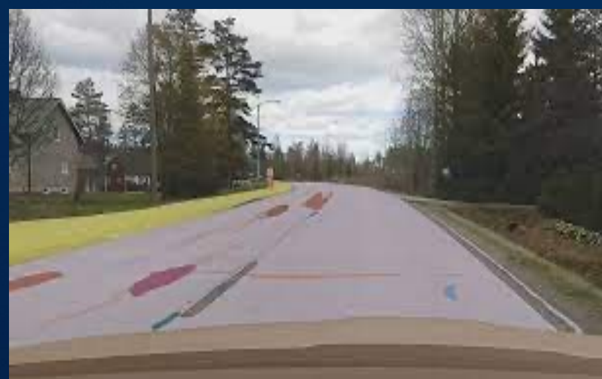
Road Condition Detection
